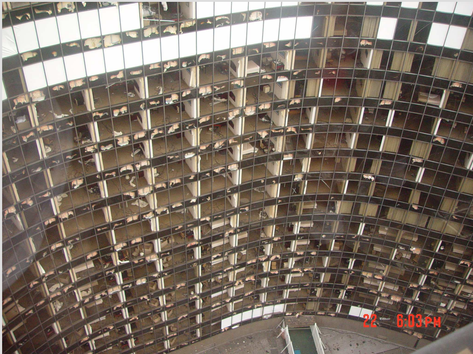
North façade of Hyatt from 1250 Poydras
