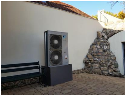
Energy efficient heating and cooling system (low-temperature air-to-water heat pump)
