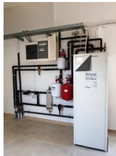
Energy efficient heating and cooling system (low-temperature air-to-water heat pump)
