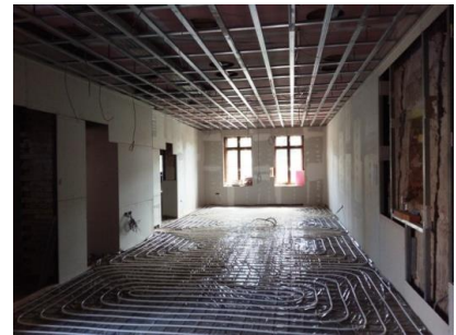
Energy efficient heating and cooling system (low-temperature air-to-water heat pump)
