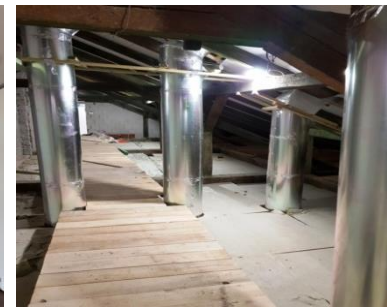
Energy efficient lighting system with Sunlite Tube System
