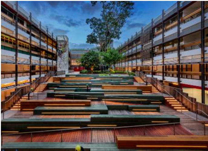
Enabling Village – 1 st integrated community space
