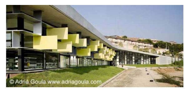
The exterior **lattice** of the north-east façade protects the reader from direct solar radiation.
